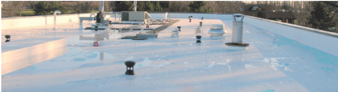
Position of VacuSeal Roof Vents are Staggered to Accommodate Variations in Wind Speed on a Completed Roof Application
