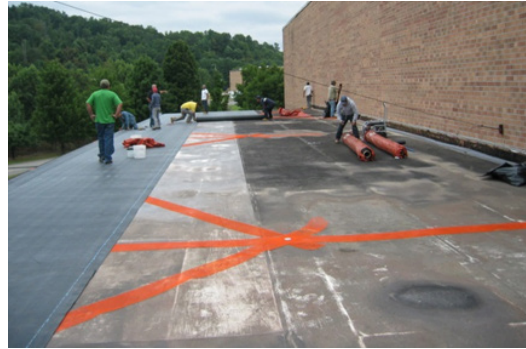
Roof Membrane is Placed Over the Distribution Strips
