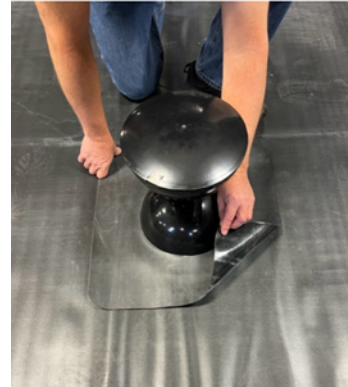
Skirt on the VacuSeal Roof Vent is Adhered Using Double-Sided Butyl Tape or hot air welded, depending on the skirt material, to the Roofing Membrane
